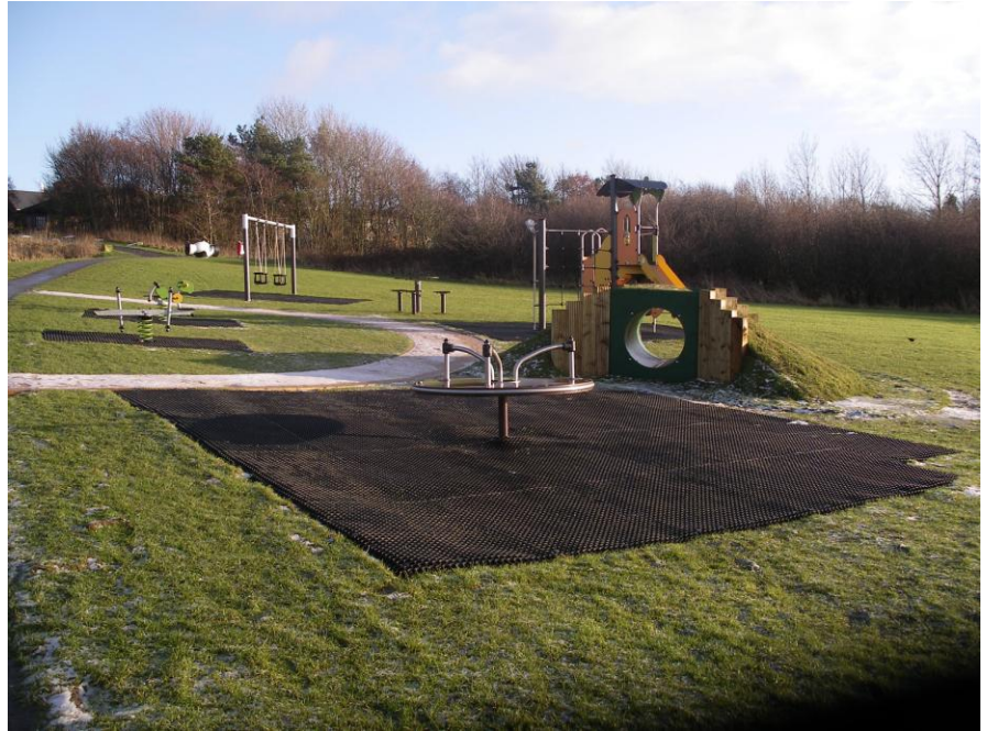
The new playground at the Millennium Green
